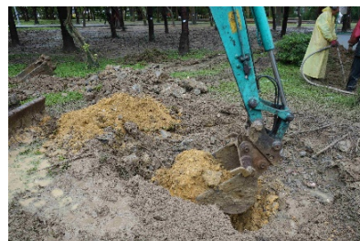
3) 挖掘代替土壤
